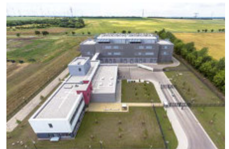
T-Systems operates Europe's most cutting-edge data center in Biere, near Saxony-Anhalt's state capital Magdeburg (© T-Systems International / Bernd Liebl)
